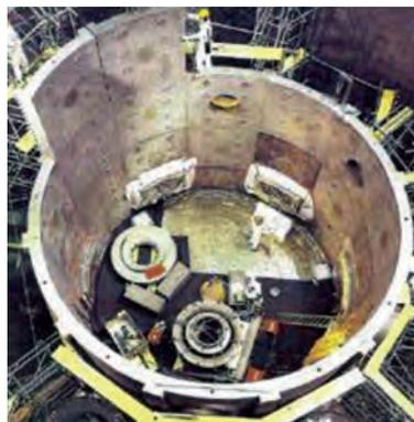
Fig. 23. Installation of the thermal shield.
