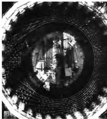
Fig. 21. Arrangement of stressing cables of the THRT-PCPV.
