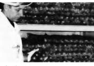
Fig. 14. Treatment of pebbes by hand, first pebble loading into the core of the AVR-HTR.
