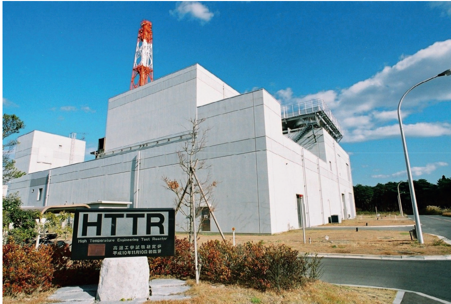
Fig. 3 External view of the HTTR building in Japan.
