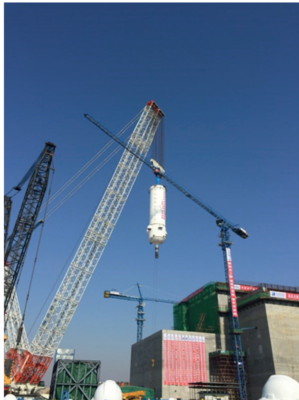
Fig. 7 Installation of RPV into HTR-PM reactor building in 2016.
